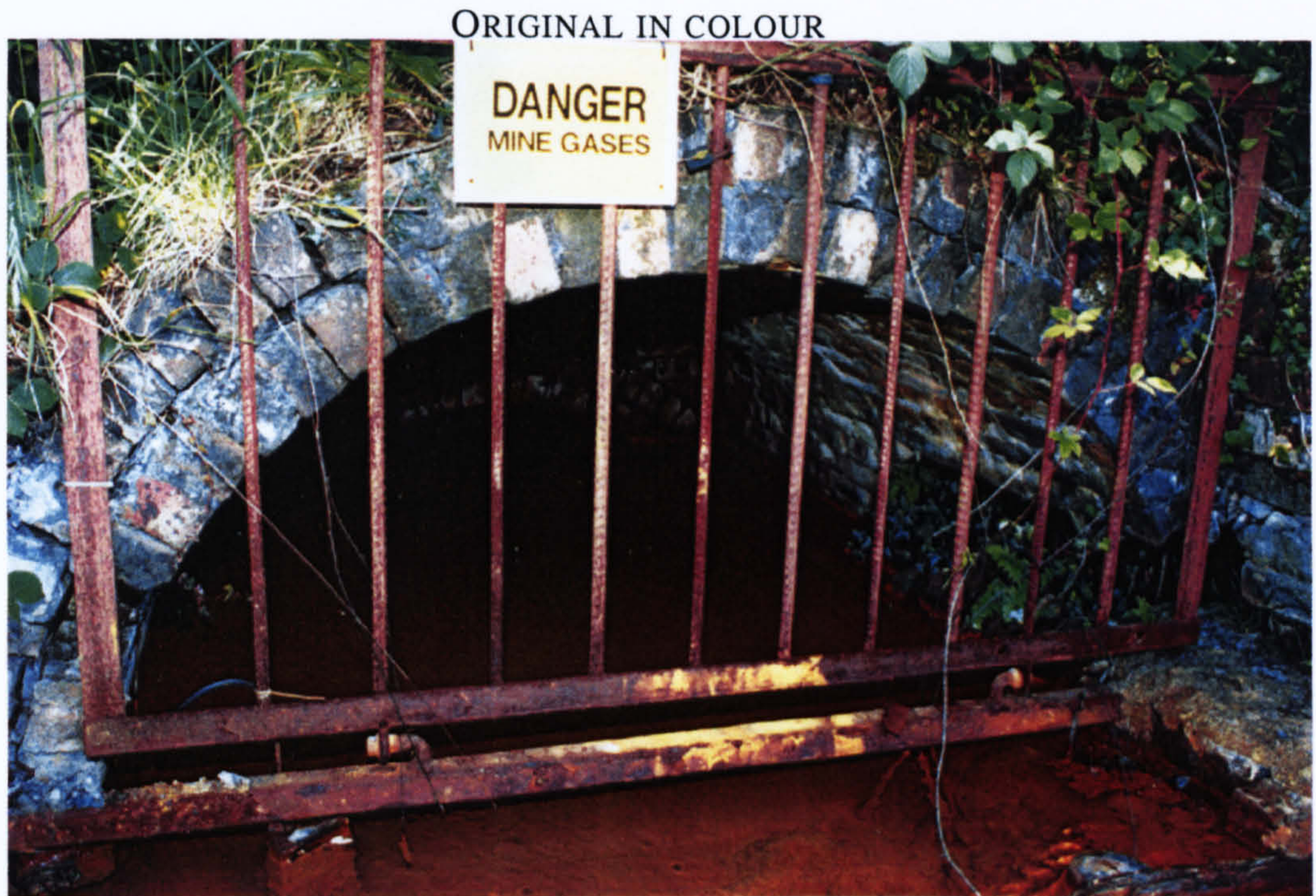
Figure 2.2: Ynysarwed mine water discharge adit.
